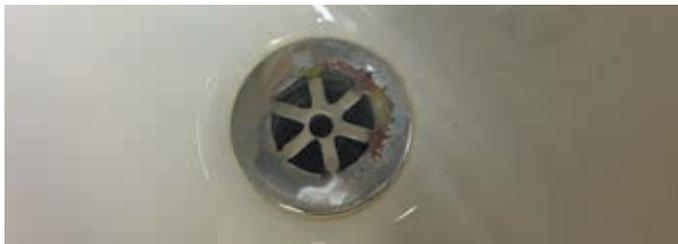
Figure 2. Example of damage to a basin plughole.
